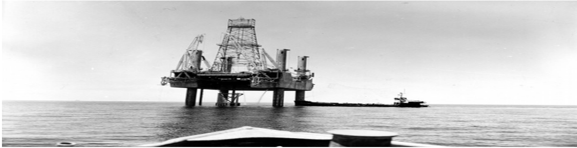
Fig. No; 11 Offshore mobile oil drilling platform in Gulf of Mexico
